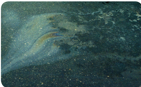
Leaking vehicle fluid can add toxic pollutants.
